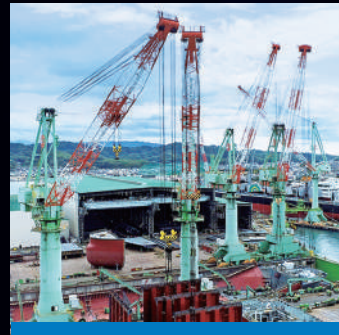
Rail Mounted Jib Crane
